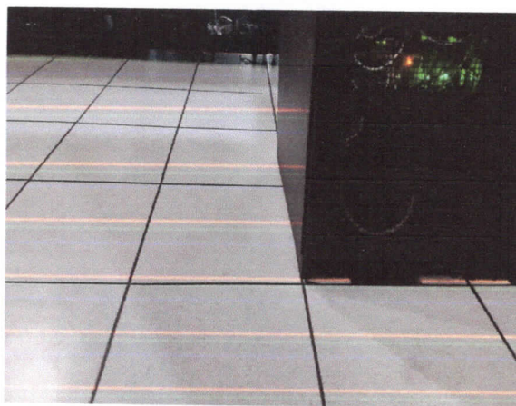
Gambar 25 Raised Floor
